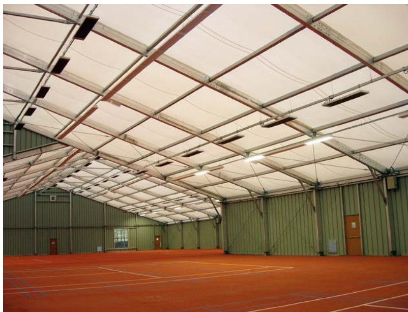
EZ300 gives instant heat and no preheating is necessary which makes it ideal for buildings that are used on an irregular basis.
