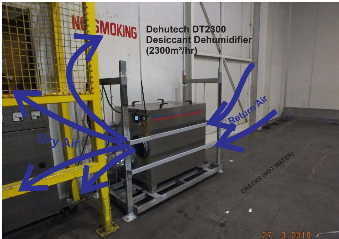
DT2300 installed in 10°C ELA Room - 3 x -25°C Freezer doors open into this room. Problem was condensation forming on ceiling, walls & wet floor, and icing in doorways - after 48 hours, no condensation or ice around the freezer doors ever since.
